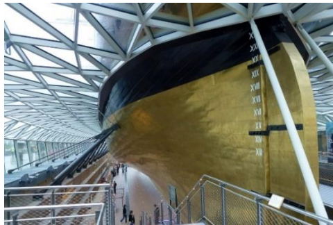
Figure 7. Cladding of ship structures with copper sheets to prevent rust and barnacles.
