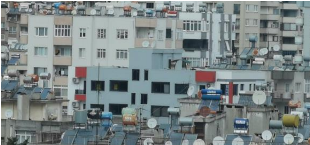
Figure 8. Solar systems and Satellite dishes competing for space on Turkish rooftops
